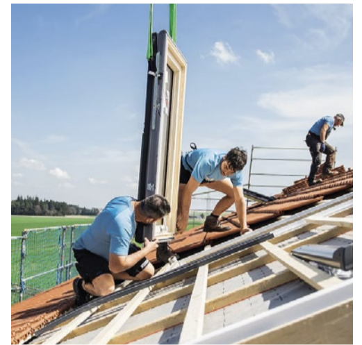
| Fabricators have a secure hold on the Designo R6 / R8 Quadro roof window as “Kurt” and “Karl” lend a hand: “Kurt” is a crane and carrying loop that is preassembled ex works and “Karl” is a perfectly compatible newly developed carry strap.
