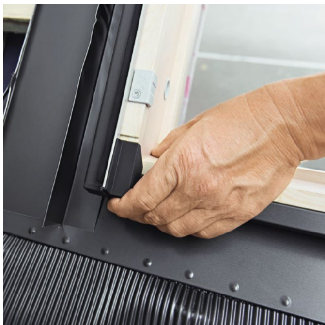
| Put in place, slide, “click”: you can hear all elements of the flashing engage, so you can be sure that installation has been completed without any errors.
